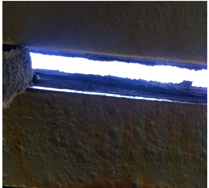
PHOTO 2 Description 18" of cs4 joint seal leakage in bay 3 over pier #5.
