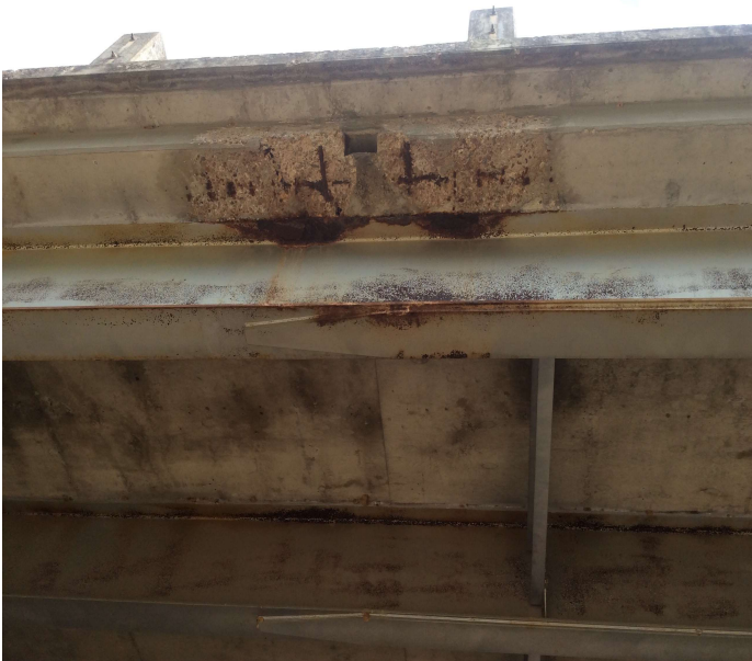
PHOTO 1 Description Typical drain spalled area
