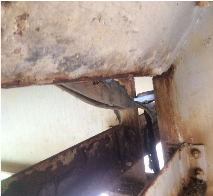
PHOTO 1 Description Dislodged joint seal typical of all locations.
